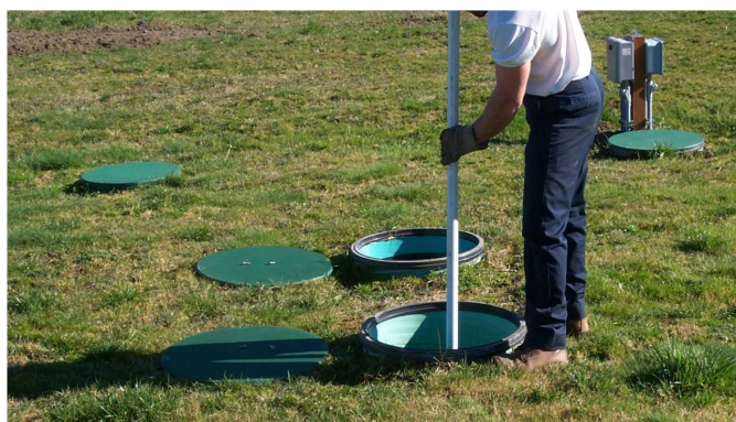
Septic Inspection in Progress
